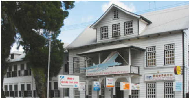
Heerenstraat. Wooden buildings are a feature of Paramaribo
