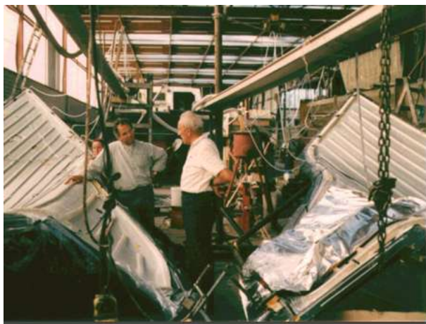
Hull construction using vacuum injection (1990)
